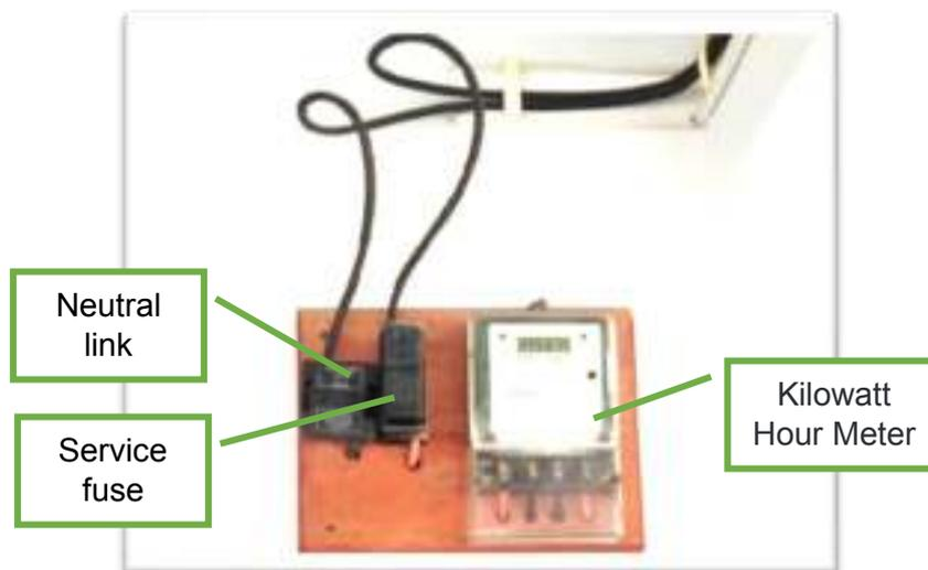
Figure 1: Service panel consists of service fuse, neutral link and Kilowatt Hour Meter
