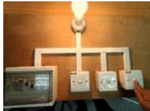
The above procedure is used to install the lighting circuit that is controlled from three points. It used two two-way switches and intermediate switch. If there is a need to control the lamp from more points or location, just add more intermediate switches in the middle of those two two-way switches. So, the lamp can be control from multiple points.
