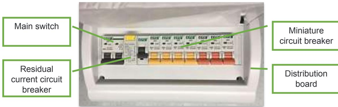
Figure 2: The main circuit consists of main switch (MS), residual current circuit breaker (RCCB) and the miniature circuit breaker (MCB).
