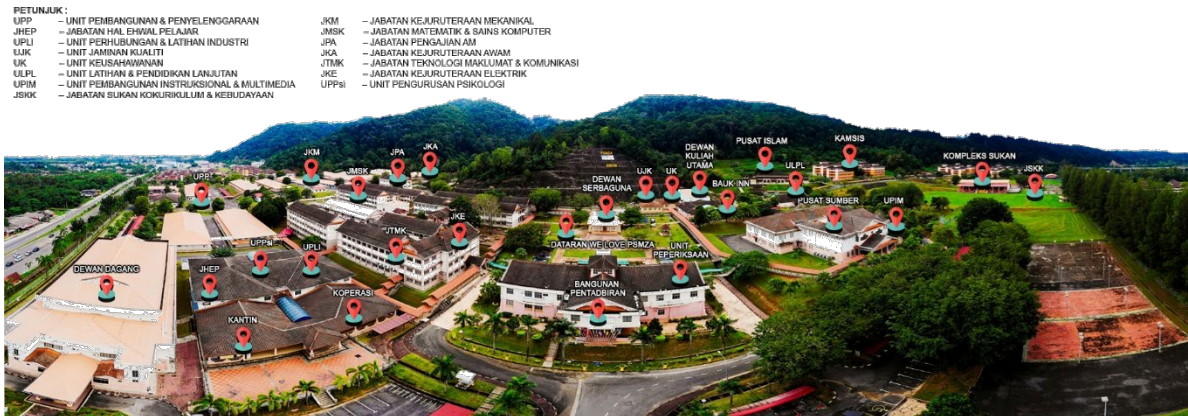
Figure 2: Aerial view of Politeknik Sultan Mizan Zainal Abidin
